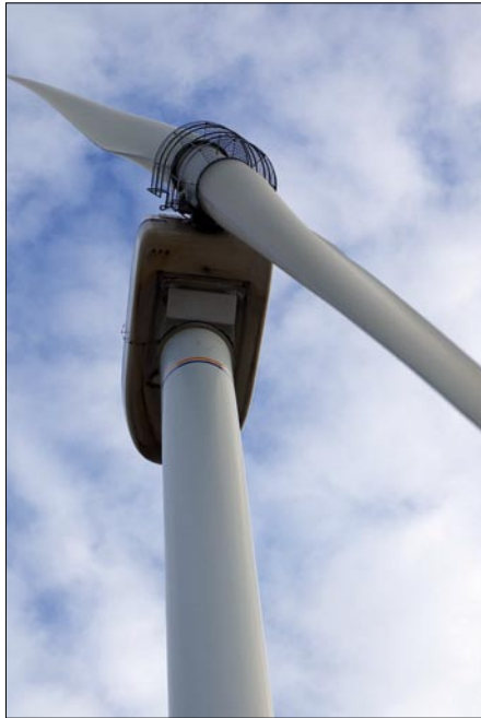
Flexible: Nordic 1 MW with two blades
